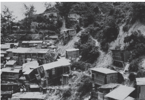
Figure 5. Landslides in 1982 affecting squatters
