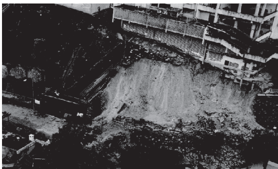
Figure 11. 1994 Kwun Lung Lau landslide
