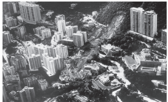
Figure 2. 1972 Po Shan Road landslide
