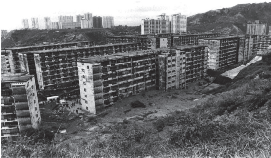
Figure 3. 1976 Sau Mau Ping landslide
