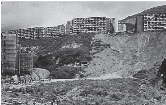
Figure 1. 1972 Sau Mau Ping landslide
