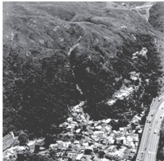
Figure 27. Debris flow at Sham Tseng San Tsuen in 1999
