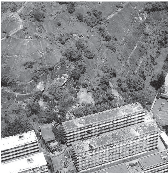
Figure 19. 1999 Shek Kip Mei landslide
